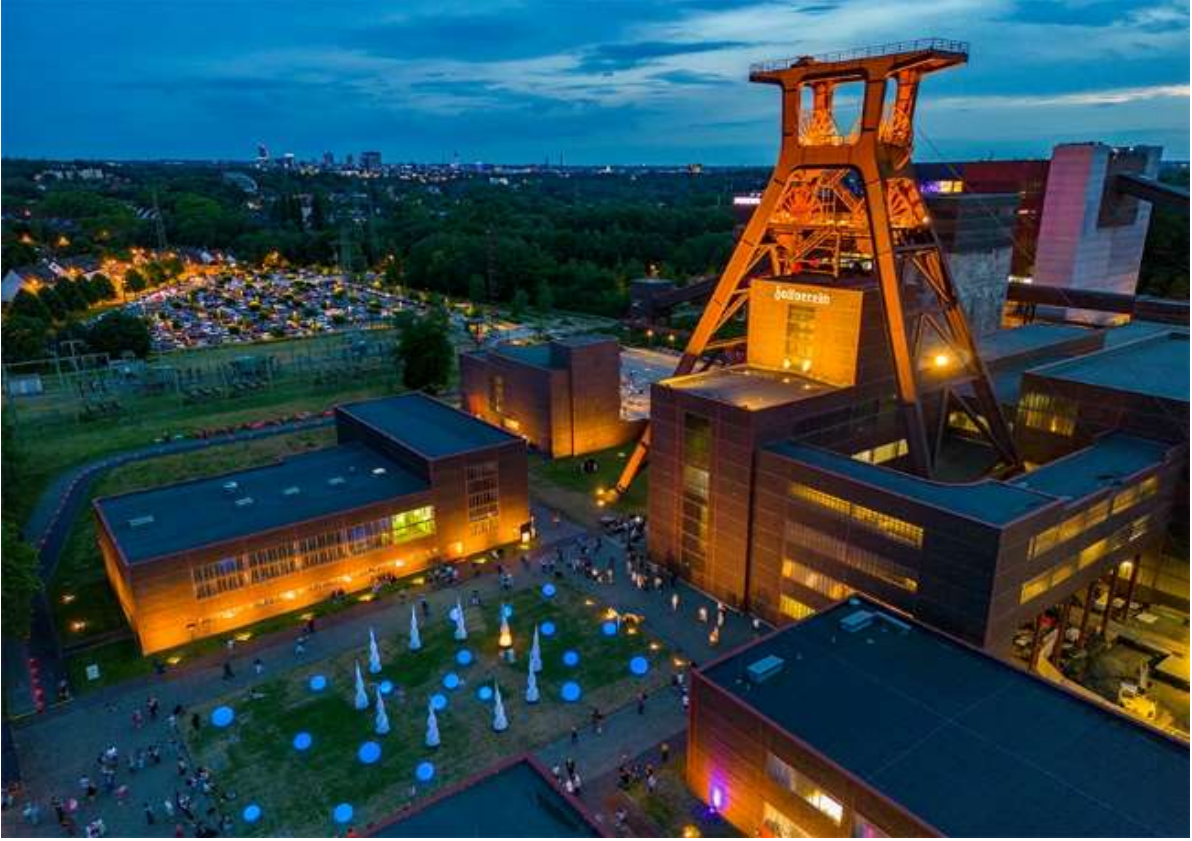
Şekil 3, Zeche Zollverein Maden Ocağı akşam perspektifi ( https://ww3.rics.org/uk/en/modus/built-environment/resilient-infrastructure/zollverein-converting-coal-mine.html ).
