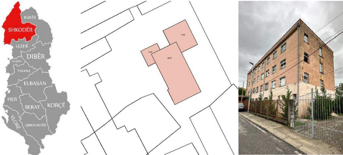
Figure 1 Location of the school in Shkoder city, Site Plan and view of the building
