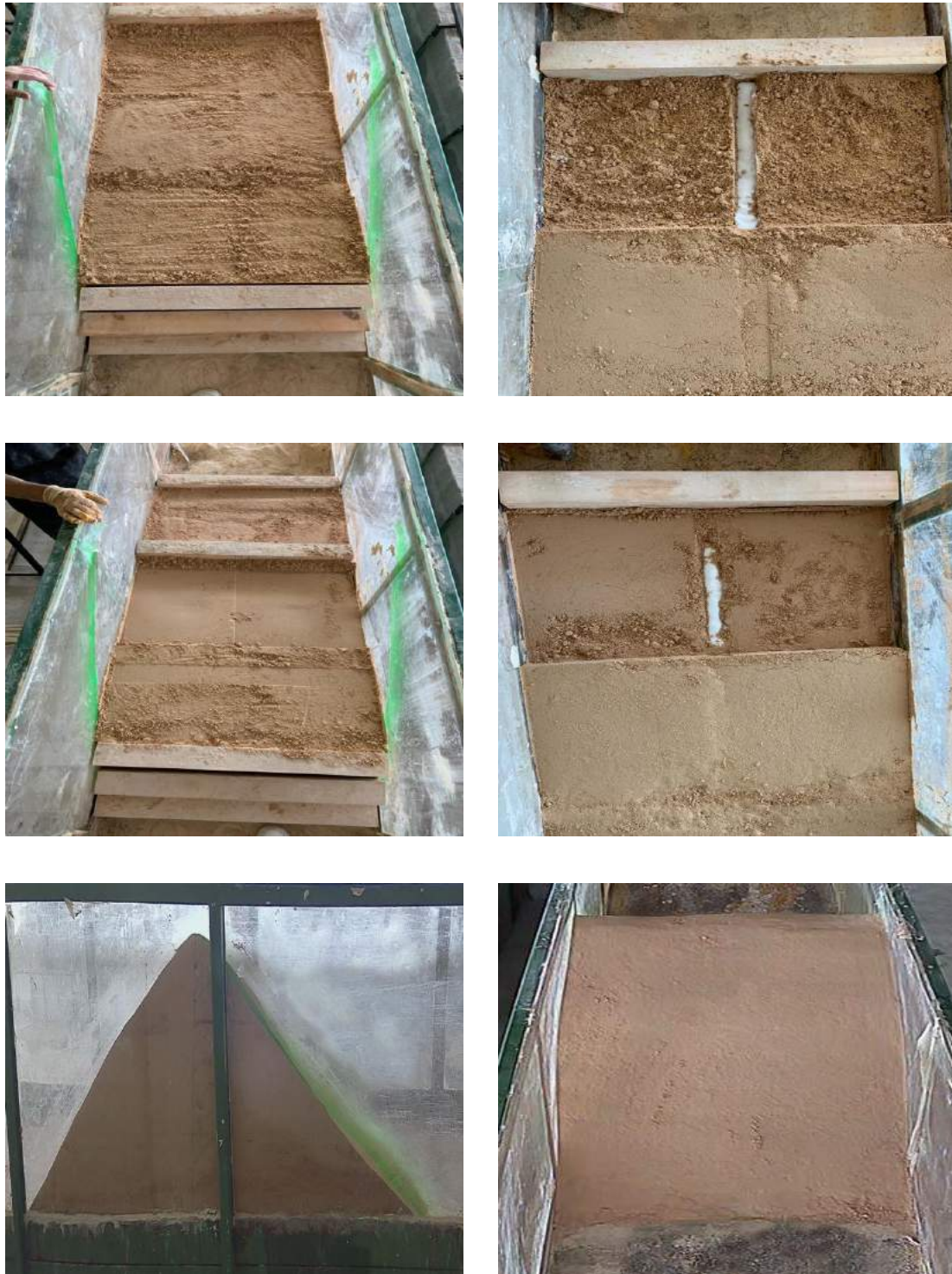
Figure 4. Some construction stages of the earth-fill dam
