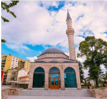
Figure 5: Iliaz Bej Mirahori mosque floor plan and front view, Korçe Source: Meksi, 2015, and author
